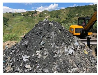
definitive executive project for the safety of the former landfill. The excavation operations of trenches are aimed at a more selective understanding of the quality of the waste present on the site: the first analyzes have highlighted the presence of waste in an advanced state of decomposition and crumbling.
